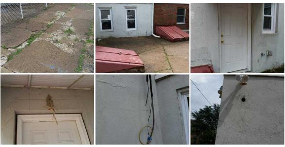
Defective City Sidewalk: Masonry - Deteriorating and damaged. A tripping hazard is
