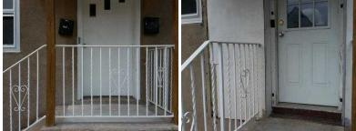
MarginalFront Walkway: Wood - Cracked and pitched towards the building.MarginalFront Entrance: Masonry - The steps are not evenly spaced and are too high.<br/>The supporting posts for the awning are improperly installed, supports bowing,<br/>and twisting and fasteners should be considered. The handrail is also detached<br/>and not secured.MarginalUtility Entrance: Masonry - Cracking skim coat.<br/>Walkway: Masonry - Cracking and deteriorating.
