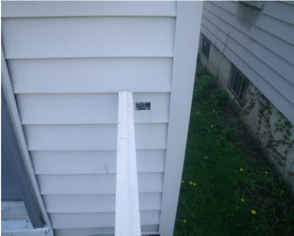
Patch hole in siding.
