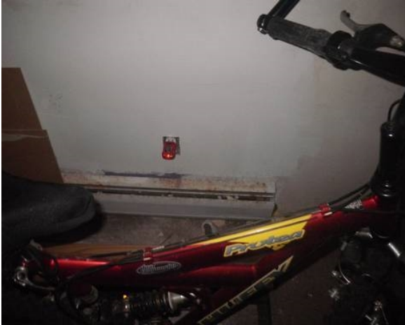
Reversed polarity.
