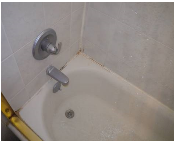
Re-caulk around tub.
