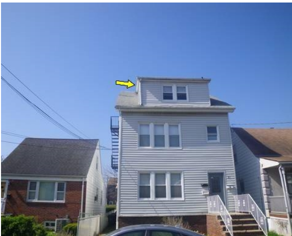
Roofline pitches down here.
