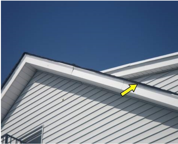
Roof appears to have 2 layers of shingles.
