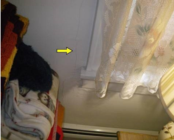
Crack near front windows tested normal for moisture.
