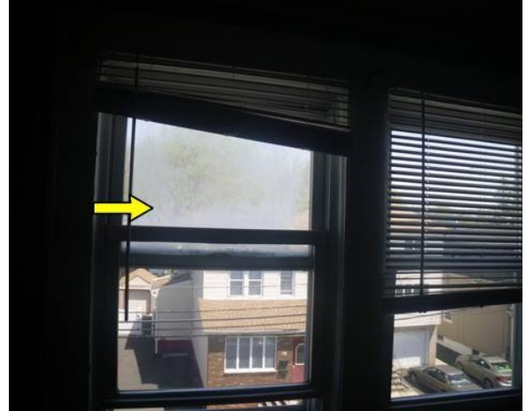
Front top window in top unit has bad seals. The other slams down if released.
