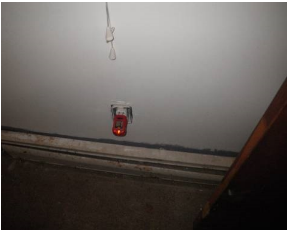
Reversed polarity.
