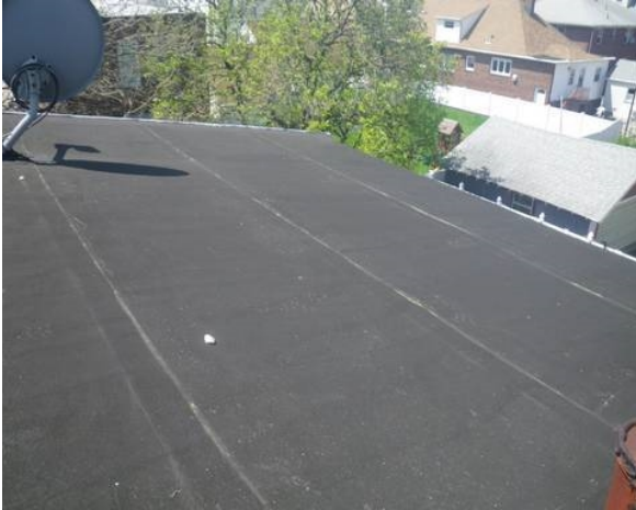
View of back low slope roof.
