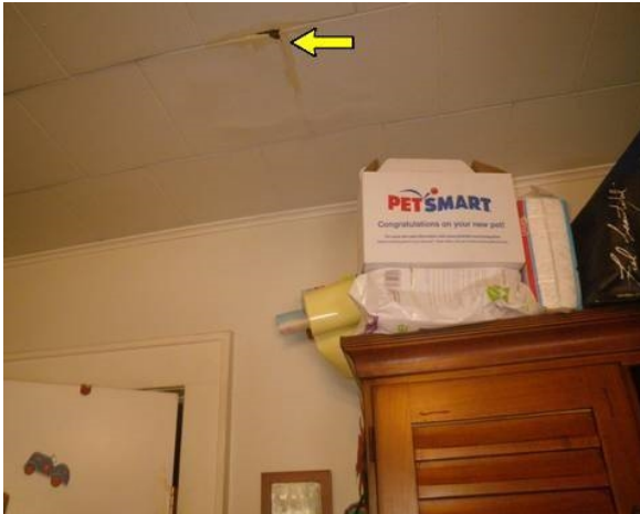
First floor dining room stained tile tested normal for moisture.
